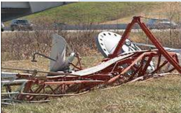
Overloaded structure
