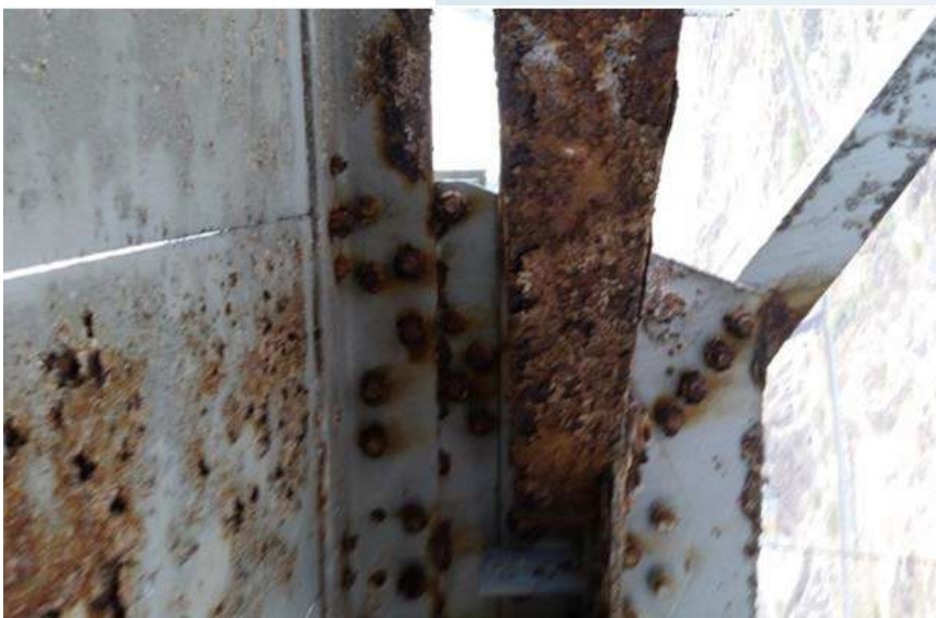
Corroded bracing
